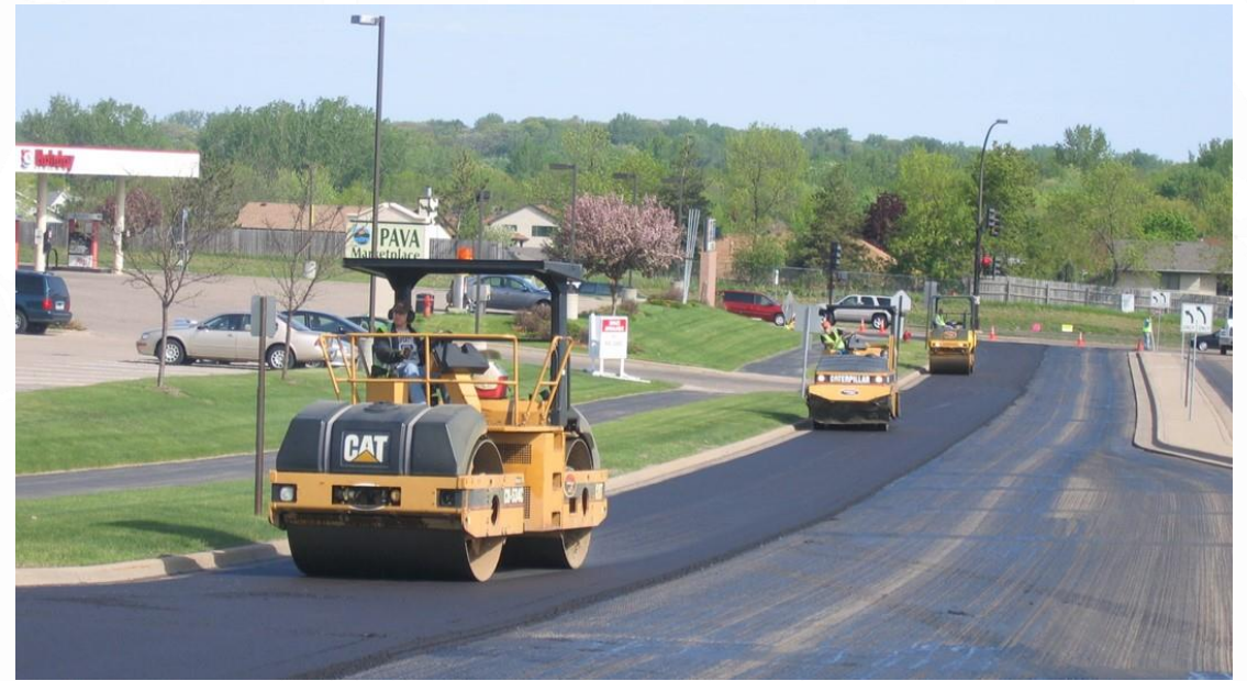
Grind and Overlay
