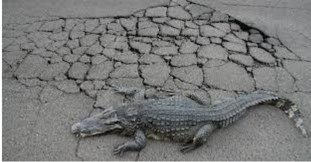
Alligator Cracking
