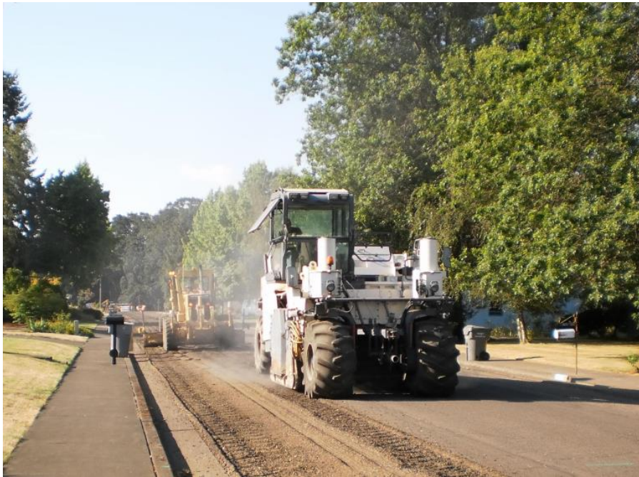
Full Depth Reclamation
