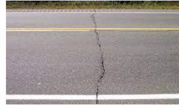
Transverse Cracking
