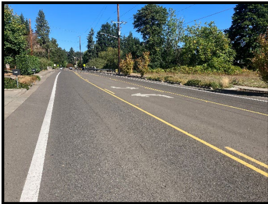
Poor Condition - PCI = 0 to 49 Del Rio Ave. west of Columbus St. – PCI = 34
