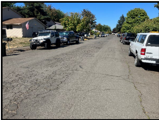
Poor Condition - PCI = 0 to 49 Del Rio Ave. west of Columbus St. – PCI = 34
