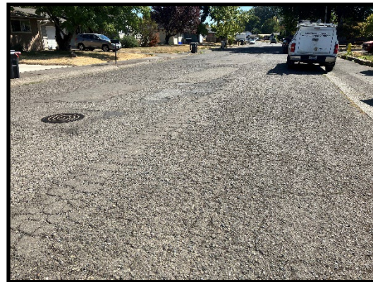
Poor Condition - PCI = 0 to 49 38th Ave. west of Thurston St. – PCI = 4
