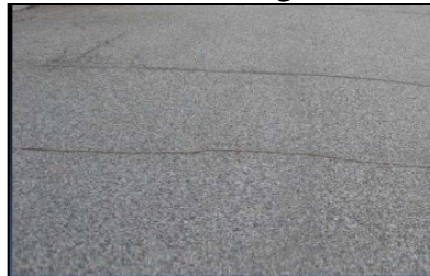
Transverse Cracking:
