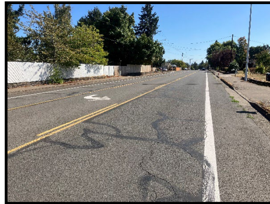
Poor Condition - PCI = 0 to 49 38th Ave. west of Thurston St. – PCI = 4
