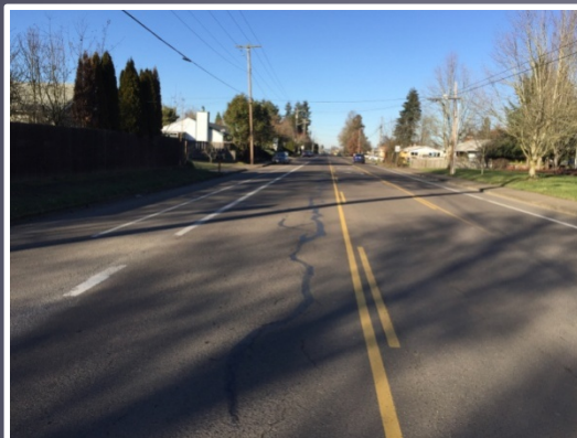
Very Poor Condition – PCI = 25 to 40 [Hill Street, 20 th -24 th Ave. – PCI = 33]
