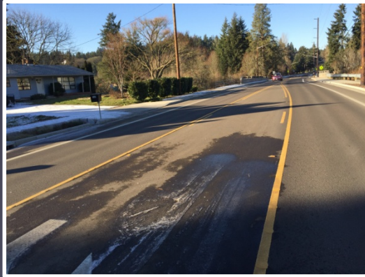
Very Poor Condition – PCI = 25 to 40 [Hill Street, 20 th -24 th Ave. – PCI = 33]
