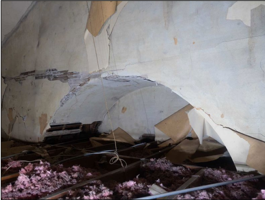
Photo 15 of 18: Interior 1892 apse arch above drop ceiling, camera facing southeast
