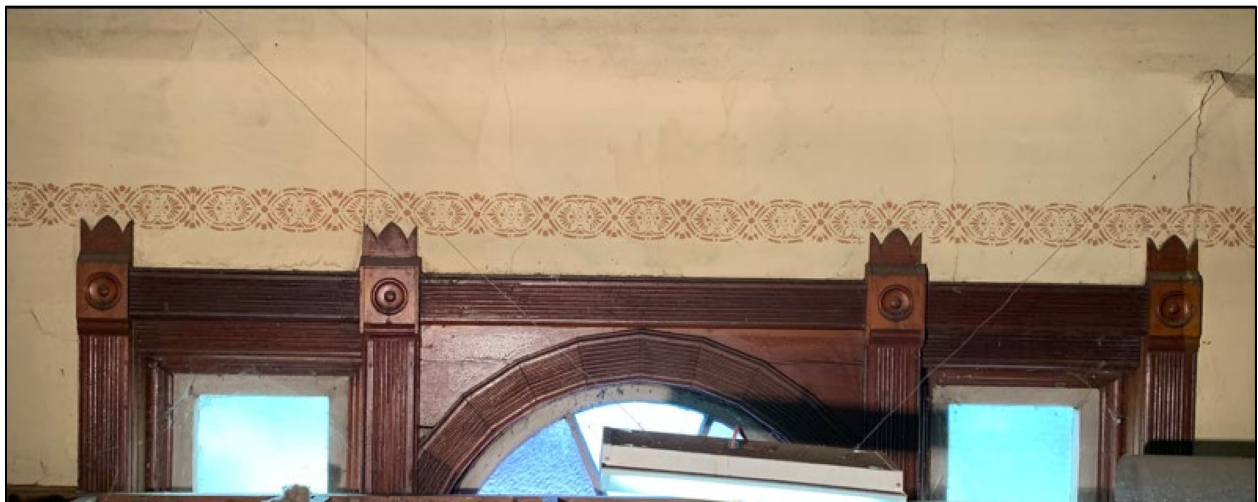
Photo 18 of 18: Interior 1892 moulding detail of ganged window in facade, camera facing north. Fluted casing topped by ornate wooden rosette style triple peaked head blocks. Copper colored wall stenciling
