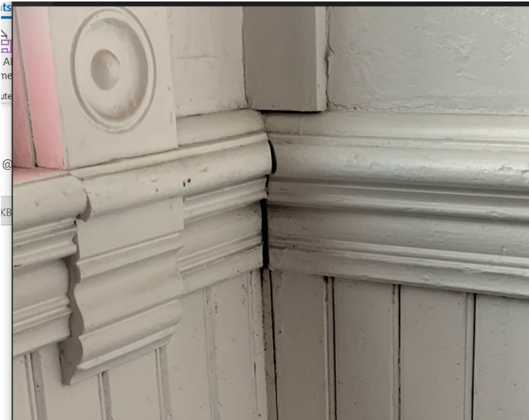
Photo 16 of 18: Interior 1892 moulding detail
