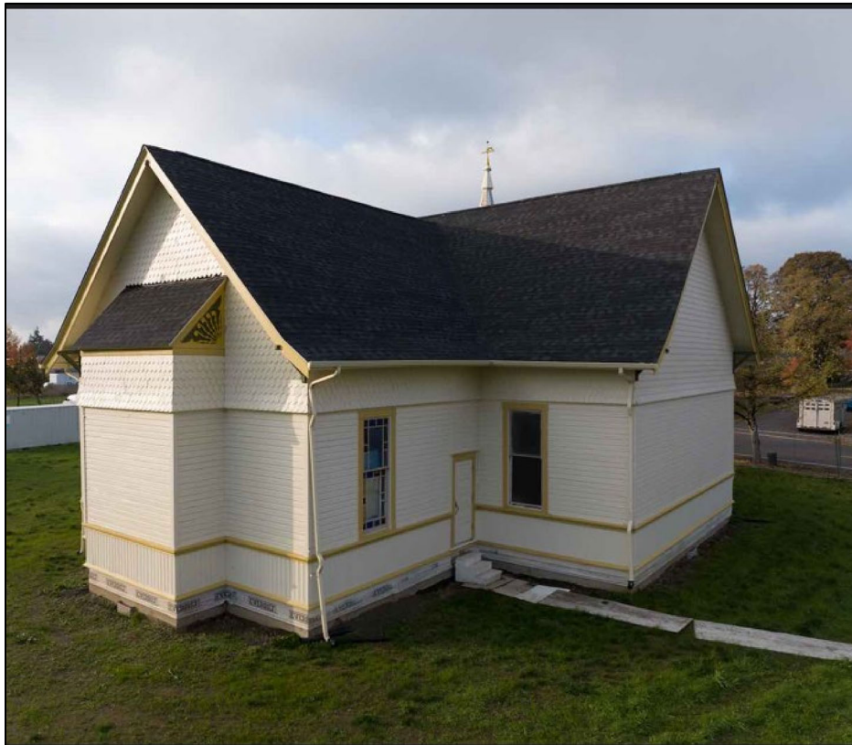
Photo 4 of 18: South elevation (left) and east elevation (right), camera facing northwest
