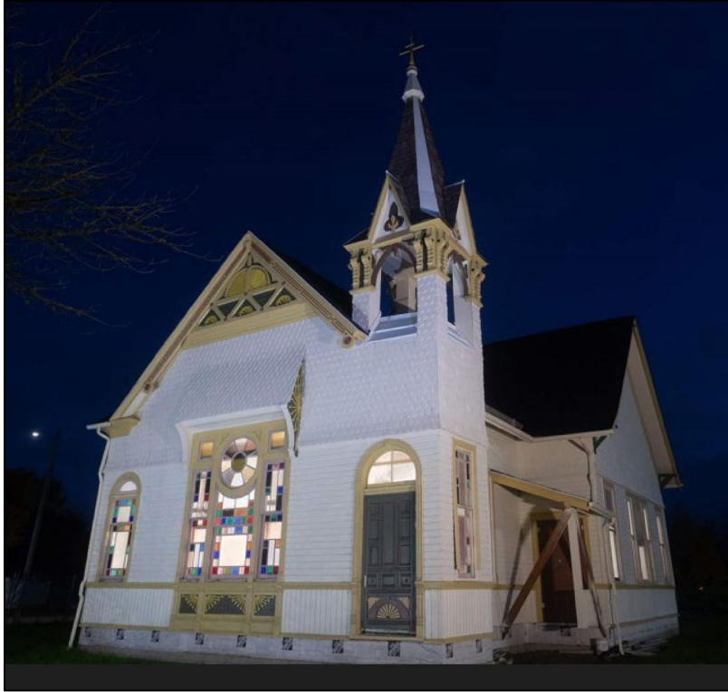
Photo 1 of 18: North façade(left) and west elevation (right), camera facing southeast
