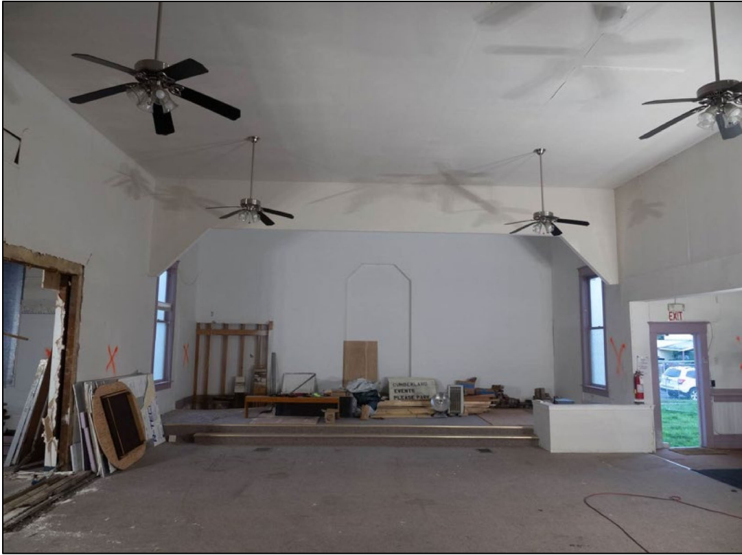
Photo 13 of 18: Interior of 1917 nave and pulpit platform, camera facing east
