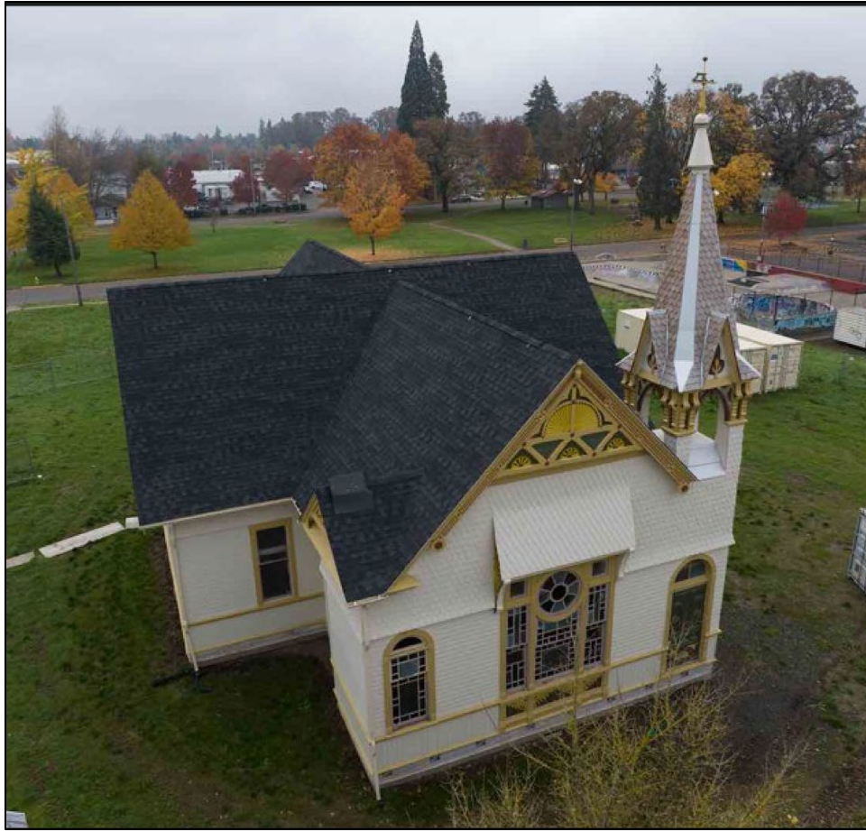
Photo 5 of 18: North façade (front) and bell tower (right), camera facing south southwest (aerial view)
