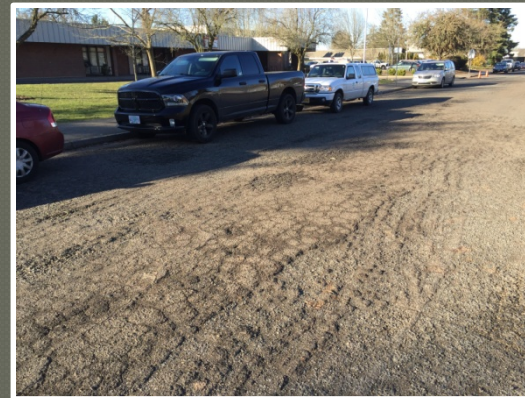
Failed Condition Streets – PCI < 10 [Oak Street at school – PCI = 5]
