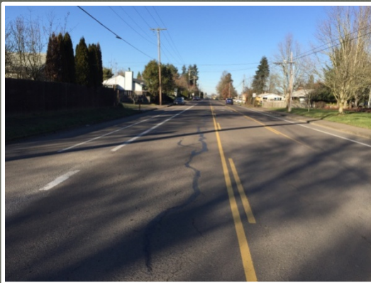
Very Poor Condition – PCI = 25 to 40 [Hill Street, 20 th -24 th Ave. – PCI = 33]
