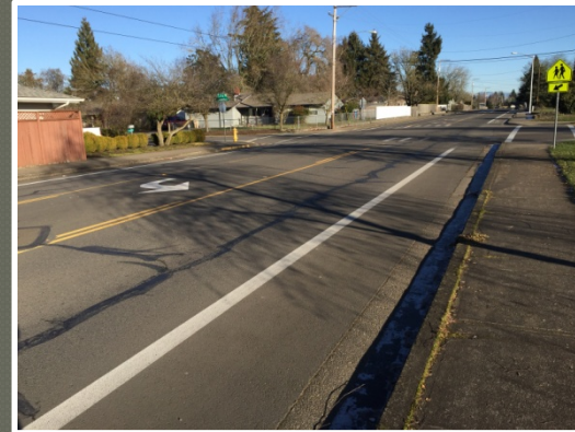
Failed Condition Streets – PCI < 10 [Oak Street at school – PCI = 5]
