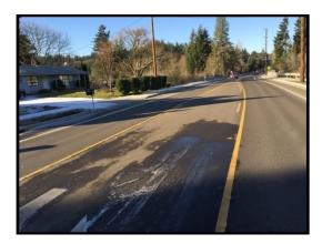
Very Poor Condition - PCI = 25 to 40[Hill Street,  $20^{th}-24^{th} \text{ Ave} - PCI = 33$ ]
