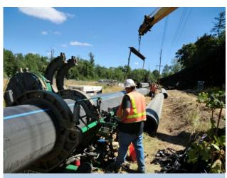
Joining 30-inch water line by heat fusion.
