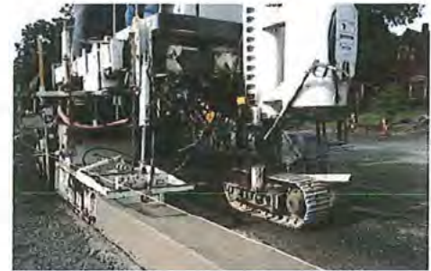
Curb installation for the Oak Street construction project.
