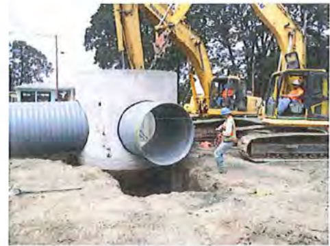
Storm drain installation in association with the Oak Street construction project.
