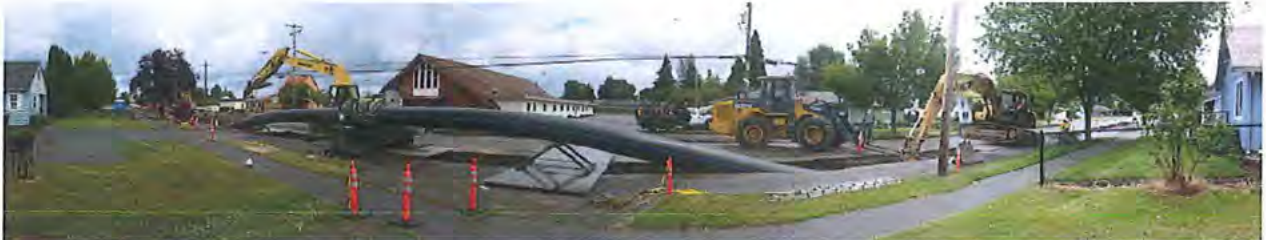
Water line construction on Hill Street.
