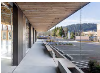
Flexible warehouse with stormwater planters and bike infrastructure integrated in parking areas
