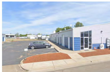
Light industrial and office building in East Albany study area
