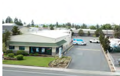
Employment areas should include sidewalks to enable employees to walk to work and generous landscape
